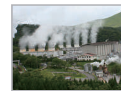
Hachobaru Power Plant (Learn about Geothermal Energy)
